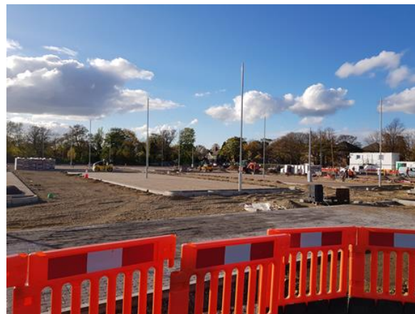
Construction of new car park
